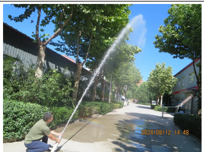
Fire hydrant testing
