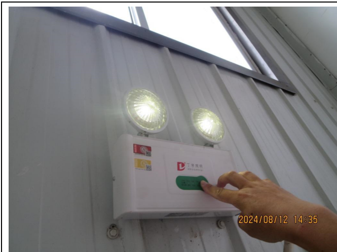
Emergency light testing
